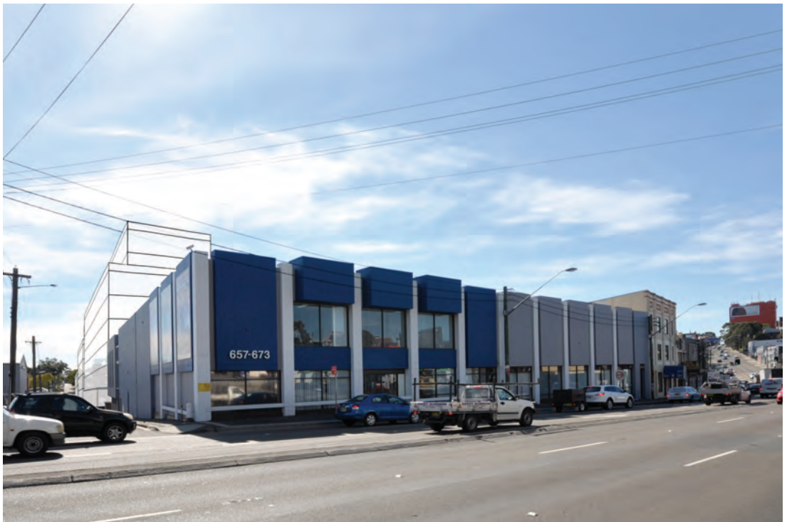
Figure 26F - View Point #5: View from Parramatta Road (cnr Upward Street), approx 100m to the South of the site
